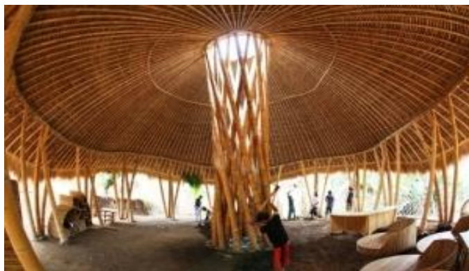
Gambar II. 18 Struktur bambu pada Green School (Sumber: http://endangerededen.wordpress.com/2009/08/26/an-ode-to-the-earths-most-sustainable-building-material-bamboo-green-school-bali/ , di akses tanggal 11 April 2014)
