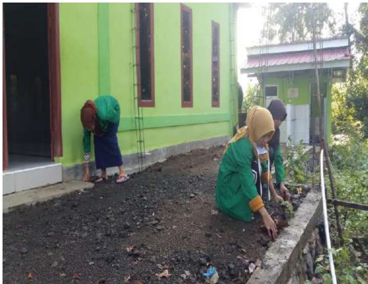
Bagian Samping Masjid Lailatul Qadri
