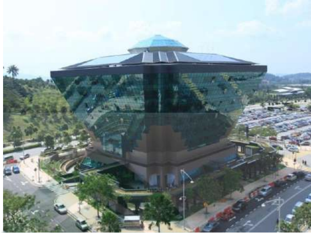
Gambar II.26. ST. Diamond building (sumber : NRarchitect, Diakses 2 mei 2016)
