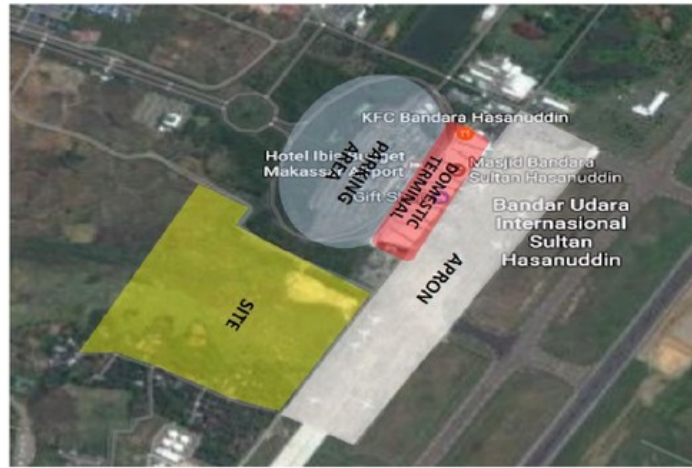
Fig. 1. Sultan Hasanuddin Airport Terminal Existing Site
