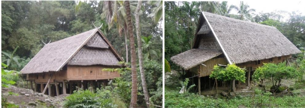
Figure 5 : Karampuang traditional house (a) Gella house (left); and (b) To Matoa house (right)
