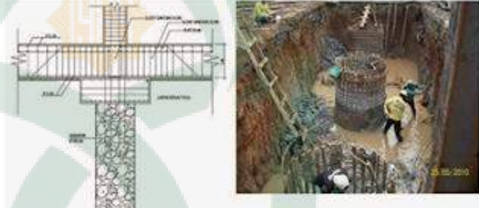
Gambar III. 37 Pondasi Sumuran
