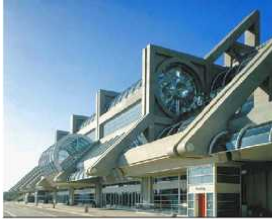
Gambar II.5 Exterior San Diego Convention Center ( http://www.aapexperience.org/ diakses 27 Mei 2015)
