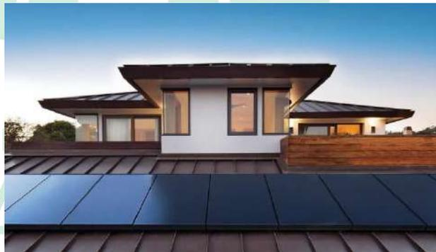
Gambar II.13 Shingle Modules PV
