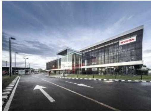
Gambar II.16. Gedung Honda Safety Riding Park Chiang Mai (Sumber: http://www.motorival.com/honda-safety-riding-park-chiangmai-tour/ , diakses pada tanggal 15 November 2018)
