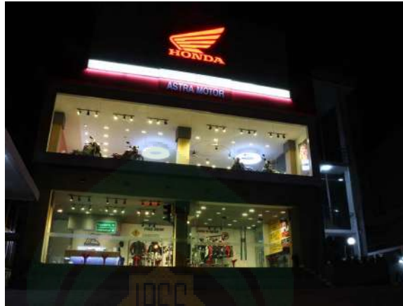
Gambar II.22. Tampak Depan Gedung Astra Motor Safety Riding Center Yogyakarta
