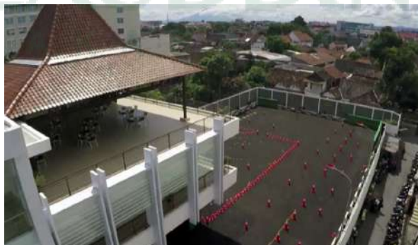
Gambar II.23. Area Belakang Gedung Astra Motor Safety Riding Center Yogyakarta
