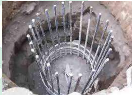
Gambar III.11 Pondasi bore pile
