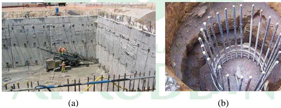
Gambar 4. 6. (a) retaining wall (b) pondasi sumuran
