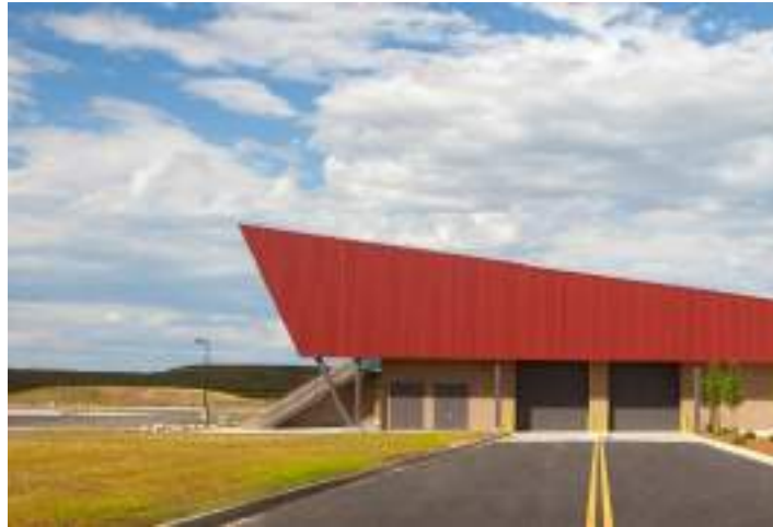
Gambar II.19 Boulder regional fire training facility (Sumber: www.archdaily.com :Roth Sheppard Architects:19 September 2011)
