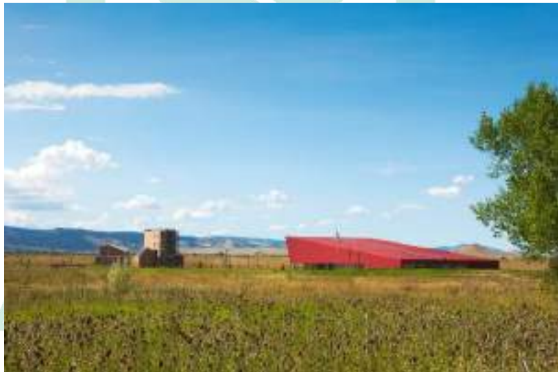
Gambar II.16 Boulder regional fire training facility (Sumber: www.archdaily.com :Roth Sheppard Architects:19 September 2011)
