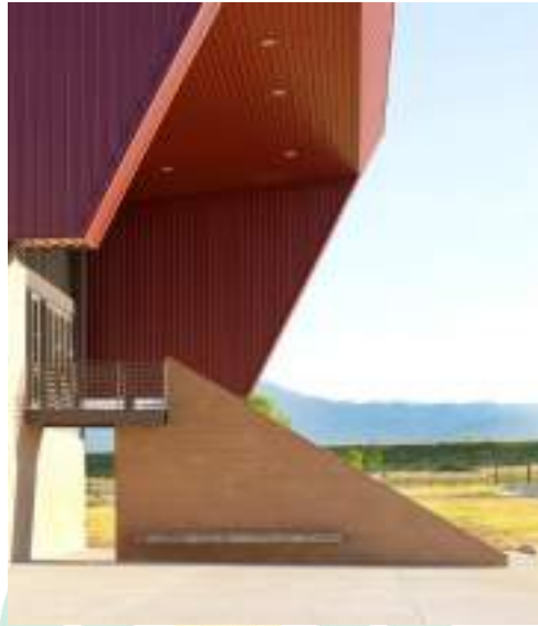
Gambar II.21 Boulder regional fire training facility (Sumber: www.archdaily.com :Roth Sheppard Architects:19 September 2011)
