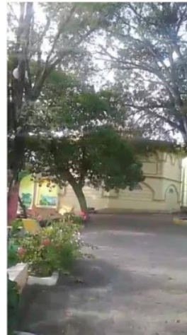
Figure 8. The wall of the mosque at 2:16
