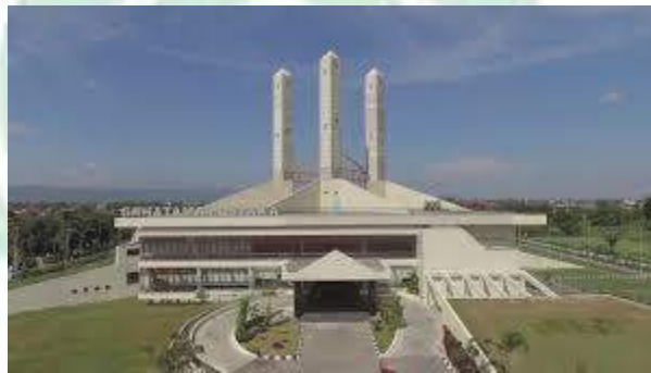
Gambar II.1 Grhatama Pustaka Yogyakarta (Sumber: Balai Yanpus DPAD DIY, 29 Jan 2017 )
