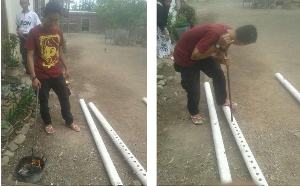
Gambar L.1: Proses Melubangi pipa paralon
