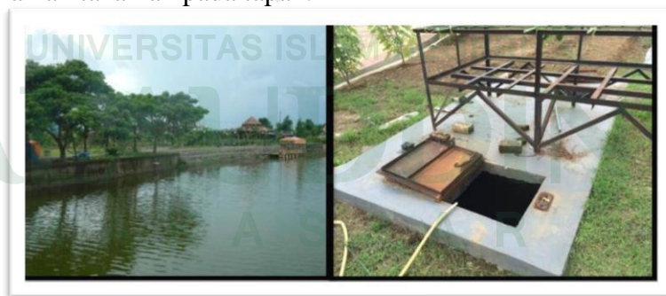
Gambar III.7 Kondisi Drainase Taman Maccini Sombala
