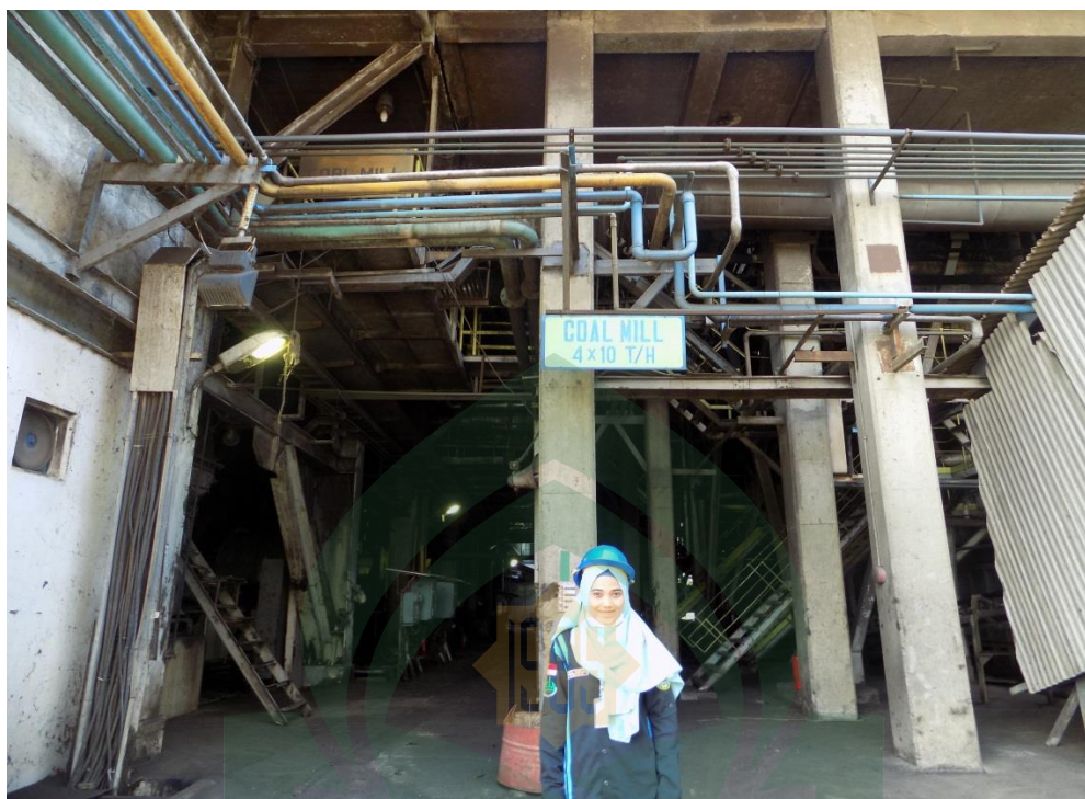
Gambar 1. BTG Power Plant 2 \times 25 MW
