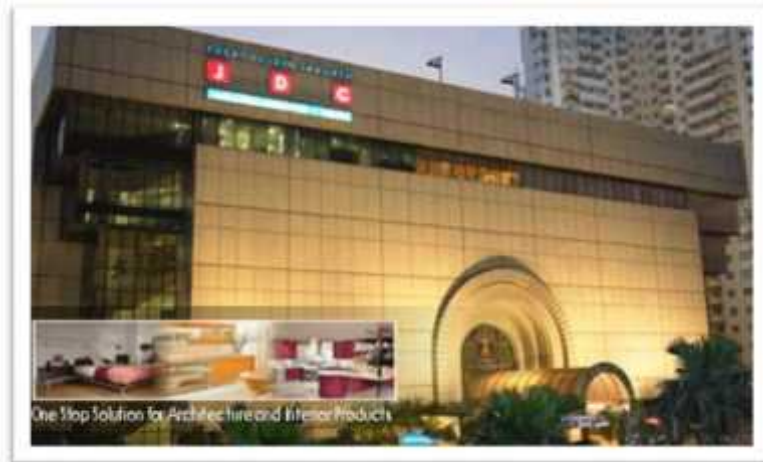
Gambar II.18. Tampak Jakarta Design Centre
